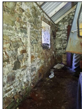
Plate 4-10 Interior section of storage shed
