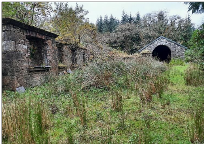
Plate 4-9 Exterior view of storage shed (right)
