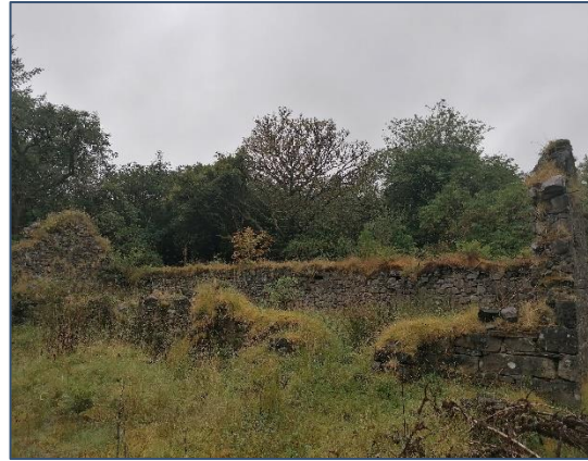
Plate 4-12 Derelict outbuilding ruins
